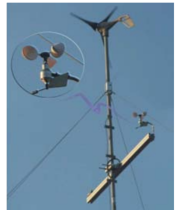
A smaller wind generator charges a battery bank in the educational unit.
