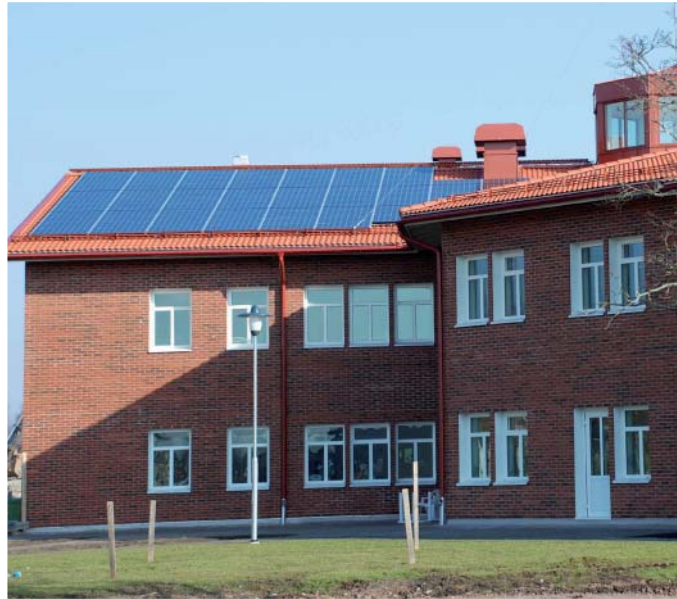
Solar cells cover 131 square meters of the school roof.
